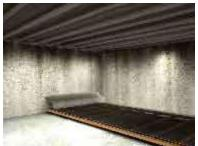
If this is new construction and you are not going to use spray foam, then it is recommended that you install a 6 mil vapor barrier on the back side of your wall studs before lifting them into position. You will also need to wrap your ceiling joists (and floor if not on slab) as shown. In some areas the local code specifies all vapor barriers must be installed on the warm side of the cellar. In those areas we highly recommend you switch to the spray foam insulation.
