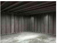
If this is a remodeling project, it is OK to wrap the existing studs in the room as shown, in a similar fashion to the ceiling joists. Make sure the vapor barrier is on the warm side of the wine cellar, meaning the exterior cellar wall.
