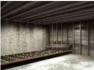
Make sure to leave excess vapor barrier at the corners so that you can wrap it, overlap the seams and tuck tape (not duct tape) them shut. Then fill all holes in studs and joists with fire rated penetration sealant to reduce air movement. Tuck Tape UV resistant adhesive is a company that sells this product. We are not recommending this company specifically, just an option so you know what you are looking for.
