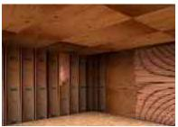
A decorative option to cover your walls and ceiling would be to apply tongue and groove material that complements the wood, stain, and/or lacquer that will be on your racking. You will first need to screw  $\hat{A}_{4}^{3}$ " marine grade plywood on your walls and ceiling so that you will be able to attach your tongue and groove.
