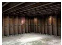
After the vapor barrier has been installed you will need to put insulation in the stud and joist cavities. The most common insulation used is fiberglass batts. In a 2x4 wall cavity using fiberglass will provide you with an R-13 insulation value. In a 2x6 wall fiberglass will
