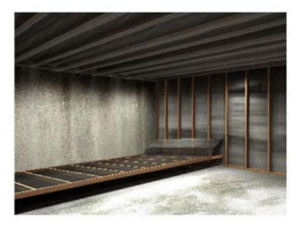
Make sure to leave excess vapor barrier at the corners so that you can wrap it, overlap the seams and tuck tape (not duct tape) them shut. Then fill all holes in studs and joists with fire rated penetration sealant to reduce air movement.
