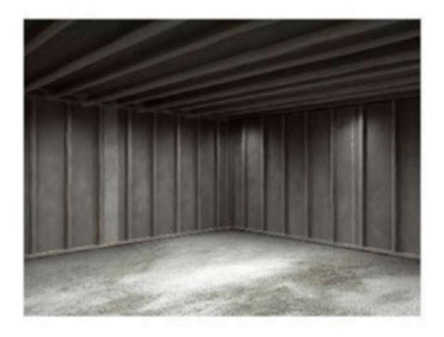
If this is a remodeling project, it is OK to wrap the existing studs in the room as shown, in a similar fashion to ceiling joists. Make sure the vapor barrier is on the warm side of the wine cellar, meaning the exterior cellar wall.
