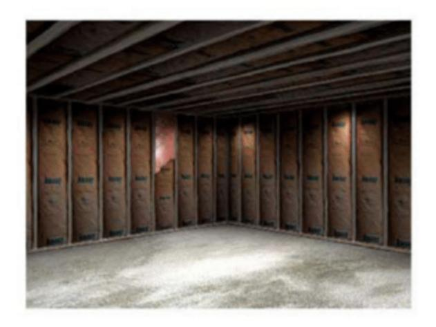
After the vapor barrier has been installed you will need to put insulation in the stud and joist cavities. The most common insulation used is fiberglass batts. In a 2x4 wall cavity, using fiberglass will provide you with an R-13 insulation value. In a 2x6 wall, fiberglass will provide you with an R-19 insulation value. The entire cavity must be "fluffed" with insulation leaving no air filled cavities.
